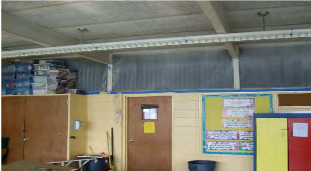
Figure 6: CONTROL CLASSROOM CEILING
