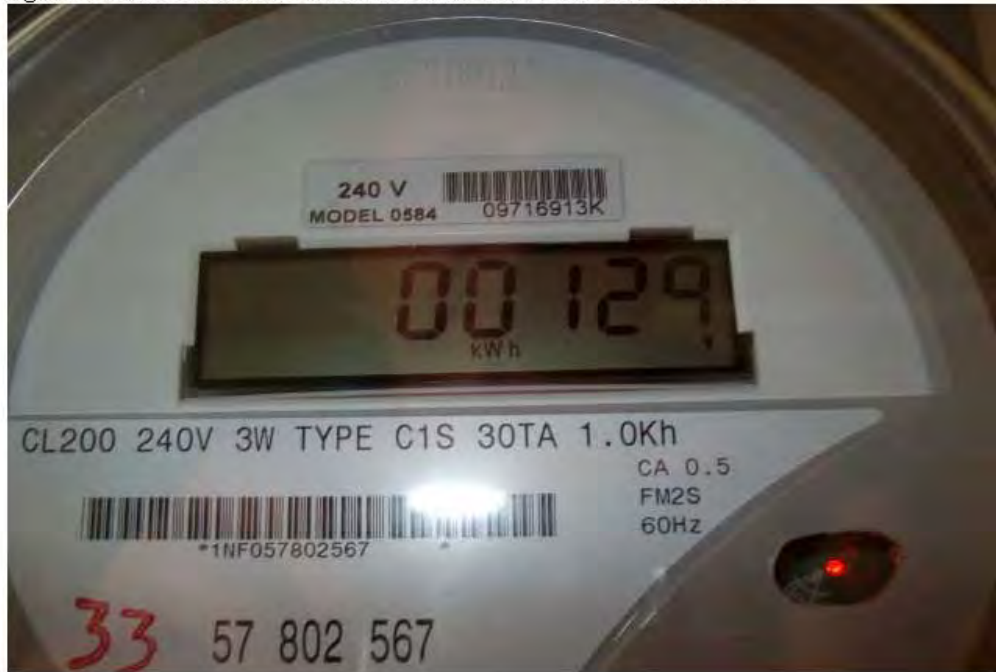
Figure 13 THIRD READING COATED ROOM 7/14/09 12:12 PM 129 KWH
