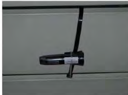
Typical Data Logger installation
