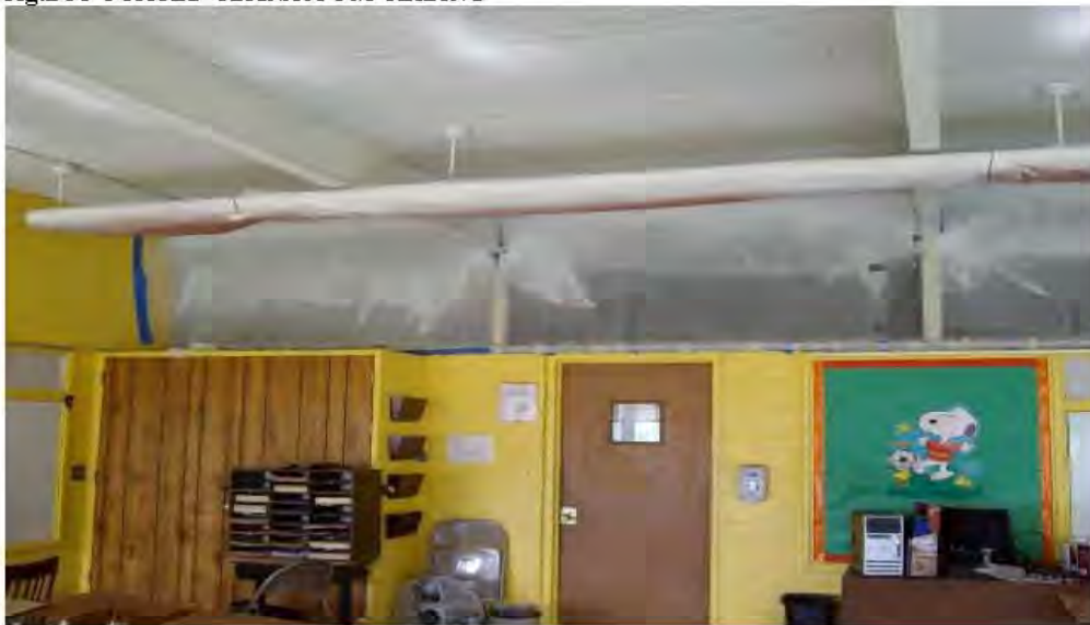
Figure 5 COATED CLASSROOM CEILING
