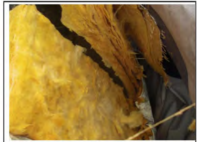
Wet insulation at unit discharge
