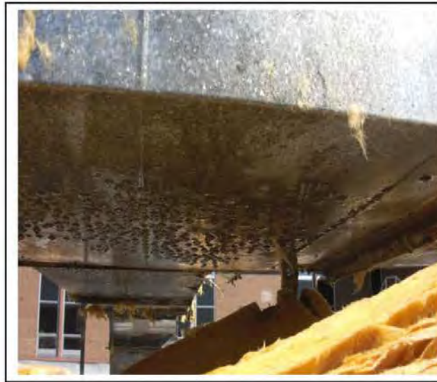
Heavv condensation droplets
