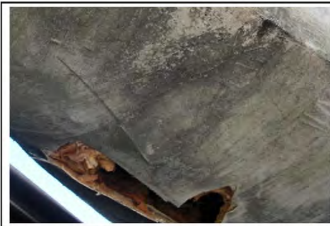
Moisture has broken through seal layer
