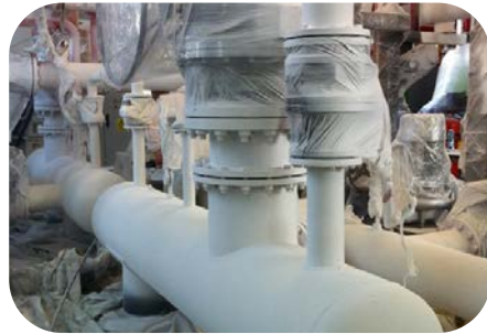
Steam pipe & valve
