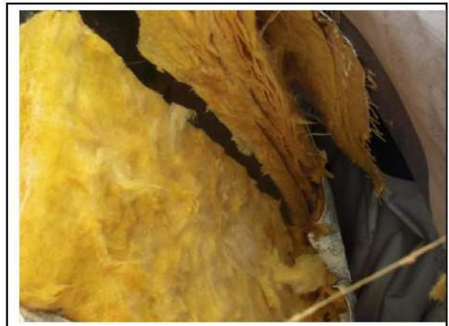
Wet insulation at unit discharge
