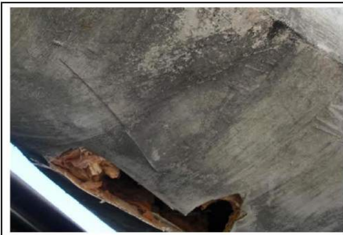
Moisture has broken through seal layer
