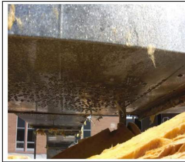
Heavv condensation droplets
