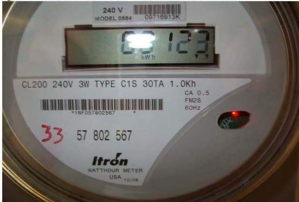
Figure 11: SECOND READING COATED ROOM 7/13/09 2:57 PM -123 KWHD
