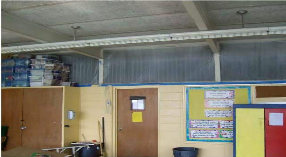
Figure 6: CONTROL CLASSROOM CEILING
