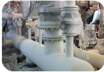
Steam pipe & valve
