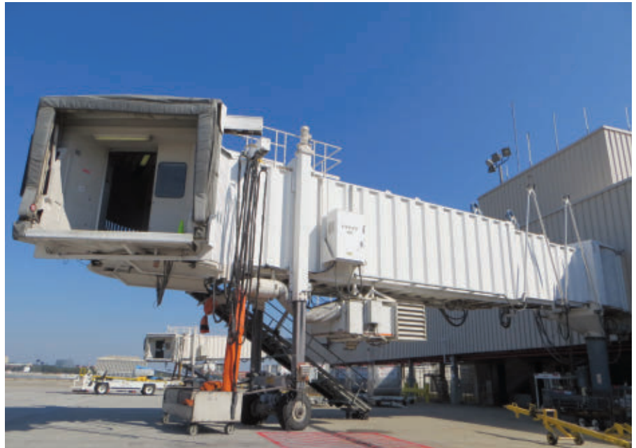
Thermal Coated Passenger Boarding Bridge at Atlanta's Gate E34
