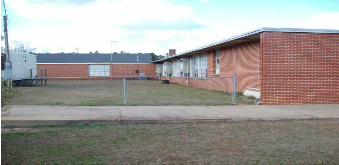
Figure 2: WEST SIDE NORTH END OF FACILITY. CLASSROOMS TESTED ARE TWO NEAREST IN PHOTO, 12 BEING THE NEAREST.
