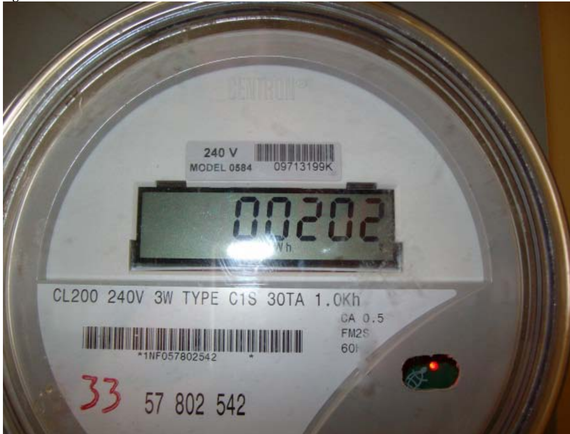
Figure 12: THIRD READING UNCOATED ROOM 7/14/09 12:13 PM 202 KWH
