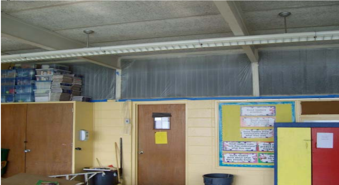
Figure 6: CONTROL CLASSROOM CEILING
