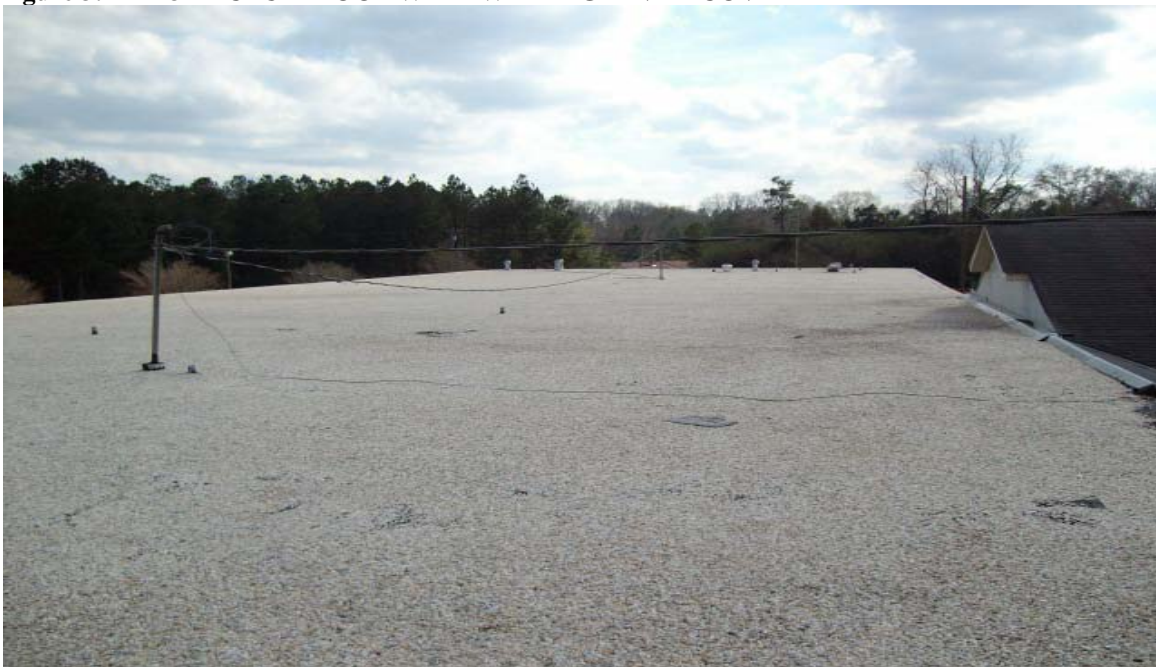
Figure 3: 2" R3 TECTUM ROOF WITH WHITE GRAVEL COVER
