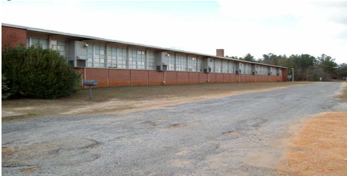
Figure 1: EAST SIDE OF FACILITY
