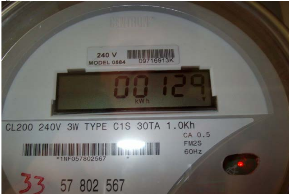
Figure 13 THIRD READING COATED ROOM 7/14/09 12:12 PM 129 KWH
