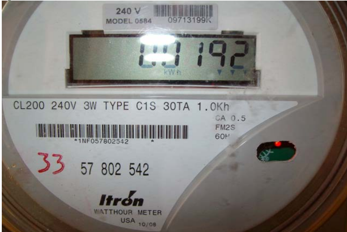
Figure 10: SECOND READING UNCOATED ROOM 7/13/09 2:58 PM – 192 KWH
