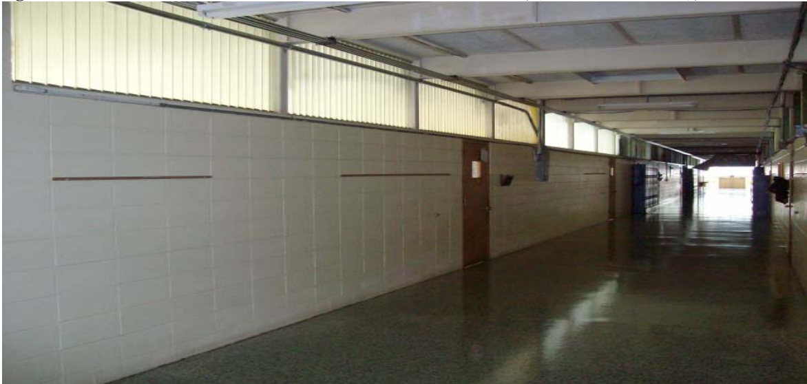
Figure 7: COMMON HALL WALL BETWEEN CLASSROOMS 12, (NEAREST DOOR), AND 11
